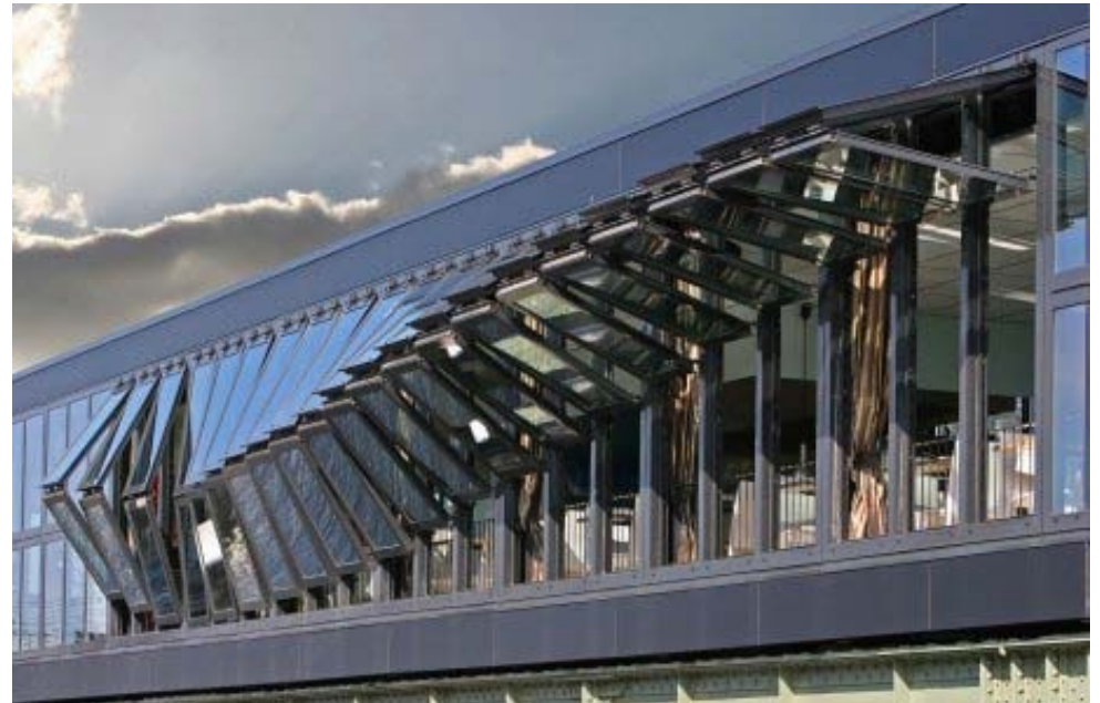
Open restaurant in Amsterdam / CIE architects
