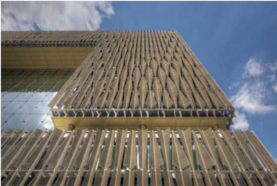
Q1 headquarters building / JSWD Architekten
